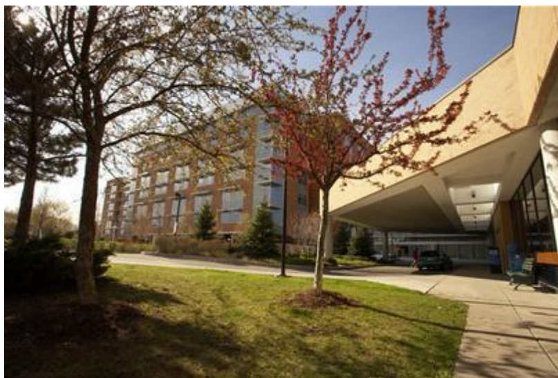
Figure 1: The Apotex Centre at Baycrest, Toronto. Website images such as this one provide a first impression to potential residents. (Source: http://www.baycrest.org/wp-content/uploads/2012/12/care-programs-01.jpg )
